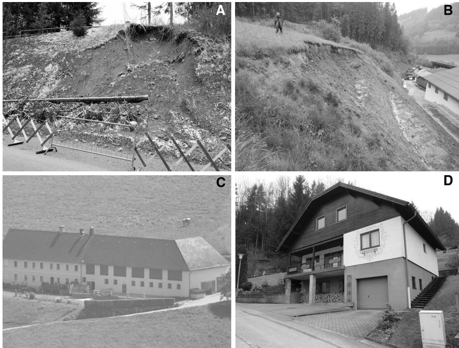
Fig. 4 Landslides affecting a street and a building in Waidhofen/Ybbs (a, b), typical farm house and a typical single family house (c, d) (pictures taken by: a Canli 2013, b, d Gokesch 2014, c Langmann/Zwirner 2011)
