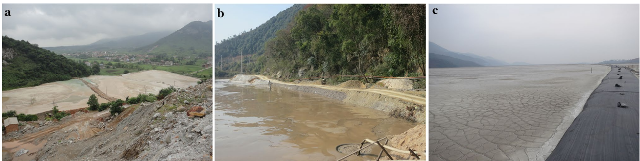
Fig. 4 Tailings sand showing the range of exit forms in ponds: a slurry; b solution; and c dried
