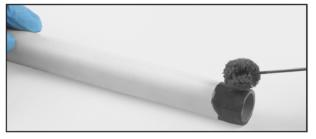
1. Apply a coat to the pipe to depth of fitting socket Work the cement into the joining surfaces using a continuous, circular motion.
