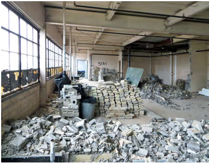
Second Floor Demolition Work
