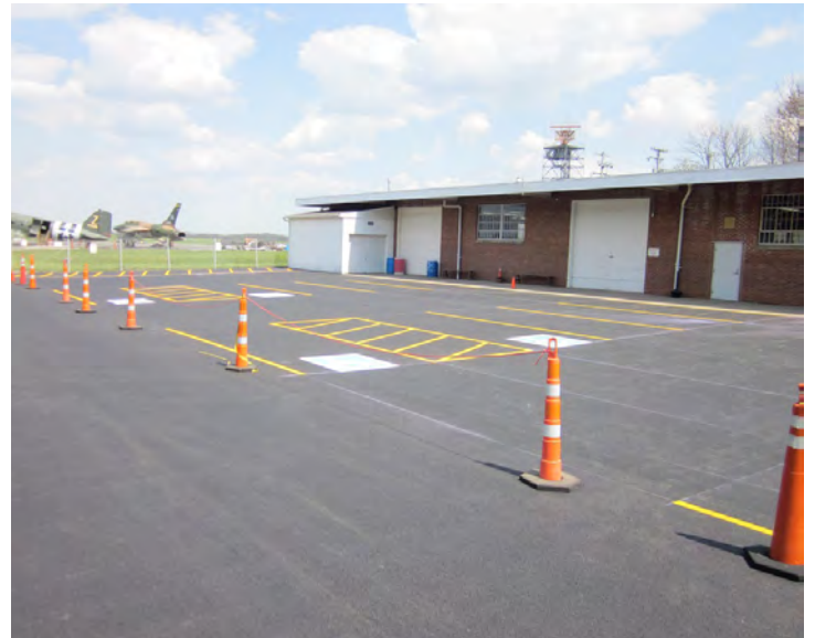
Parking Lot Upgrade
