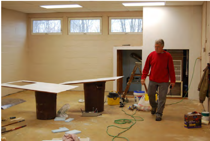
Museum Office Construction
