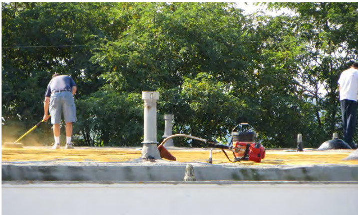
Restoration Roof Replacement
