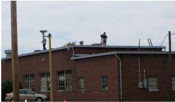
Motor Pool Roof Replacement
