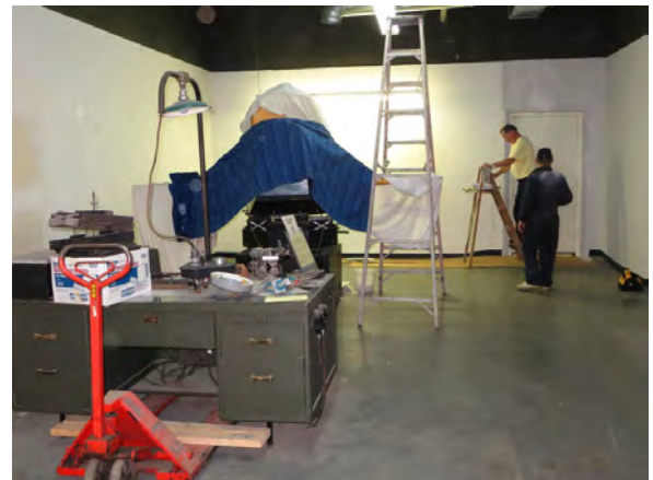
Break Area Construction
