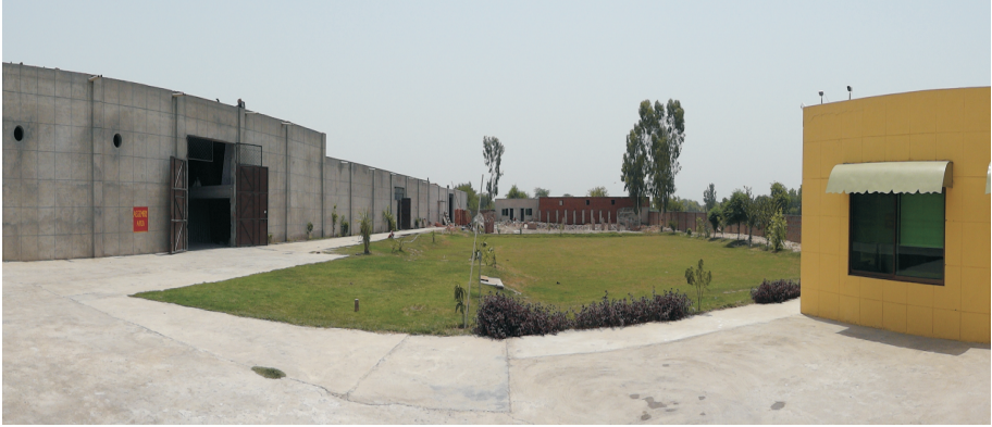
A View of our Production Plant
