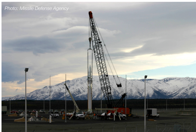
A GBI is lowered into its silo in Fort Greely, Alaska in 2004
