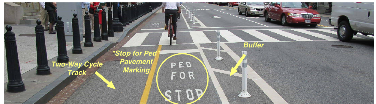
Figure 8. Two-way cycle track near F Street intersection.
