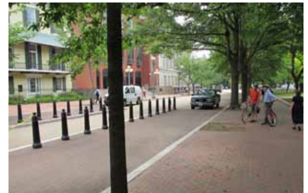
The Whitehouse Plaza area along the 15 th Street cycle track.
