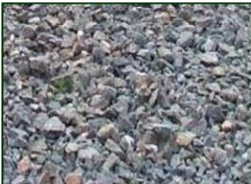
Ballast rock surface
