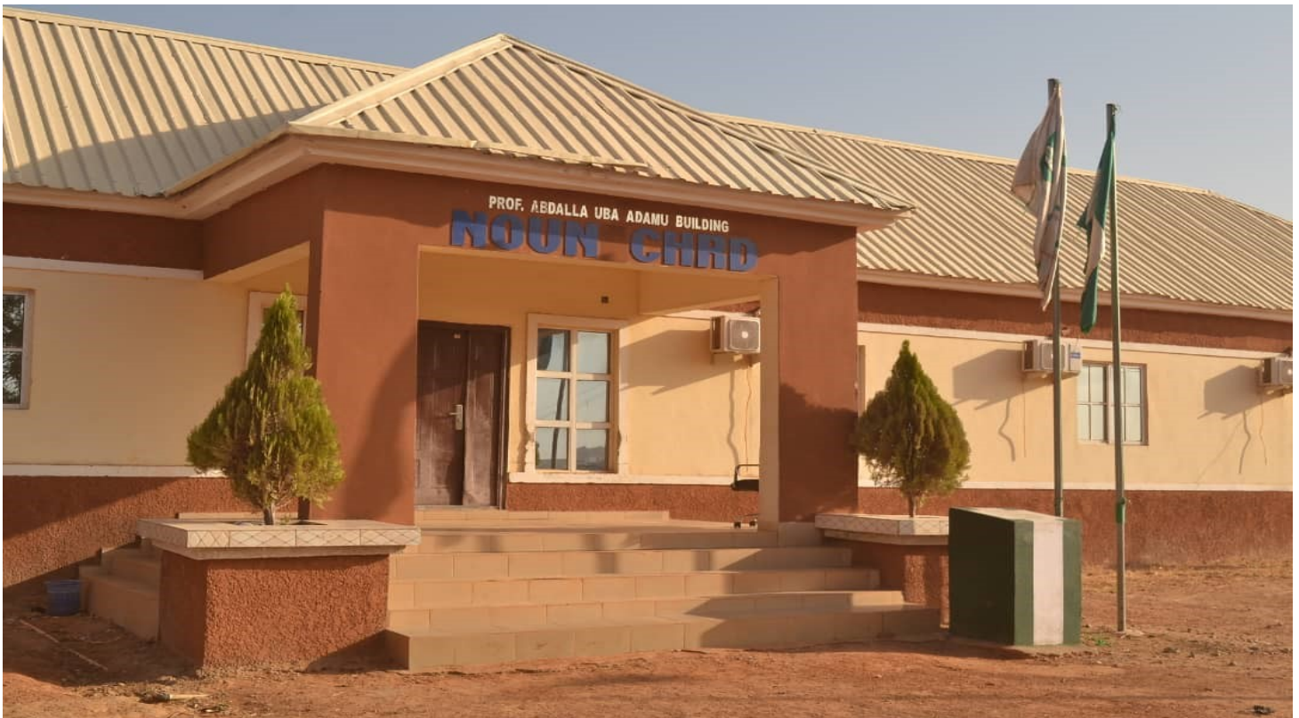
Front view of the Centre for Human Resources Development, Kaduna at Rigachikun, Kaduna
