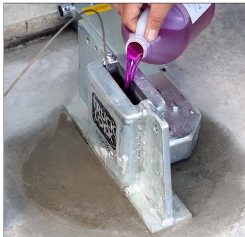
Routine maintenance for the NOVA Truck Lock™ Vehicle Restraint requires replacing the Juice-E fluid annually
