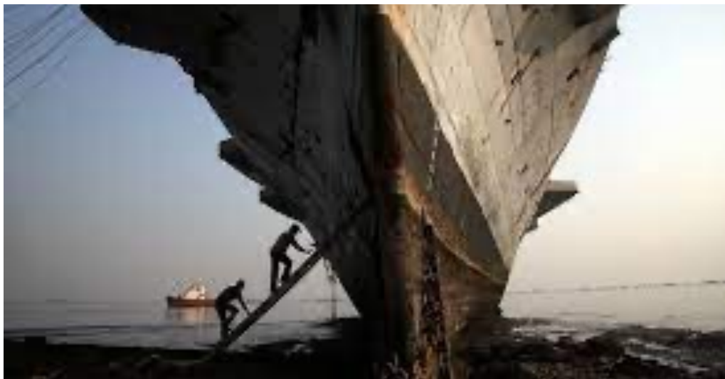
Figure 24: Ship breakers – Courtesy of https://www.theatlantic.com/photo/2014/11/the-ship-breakers/100859/
