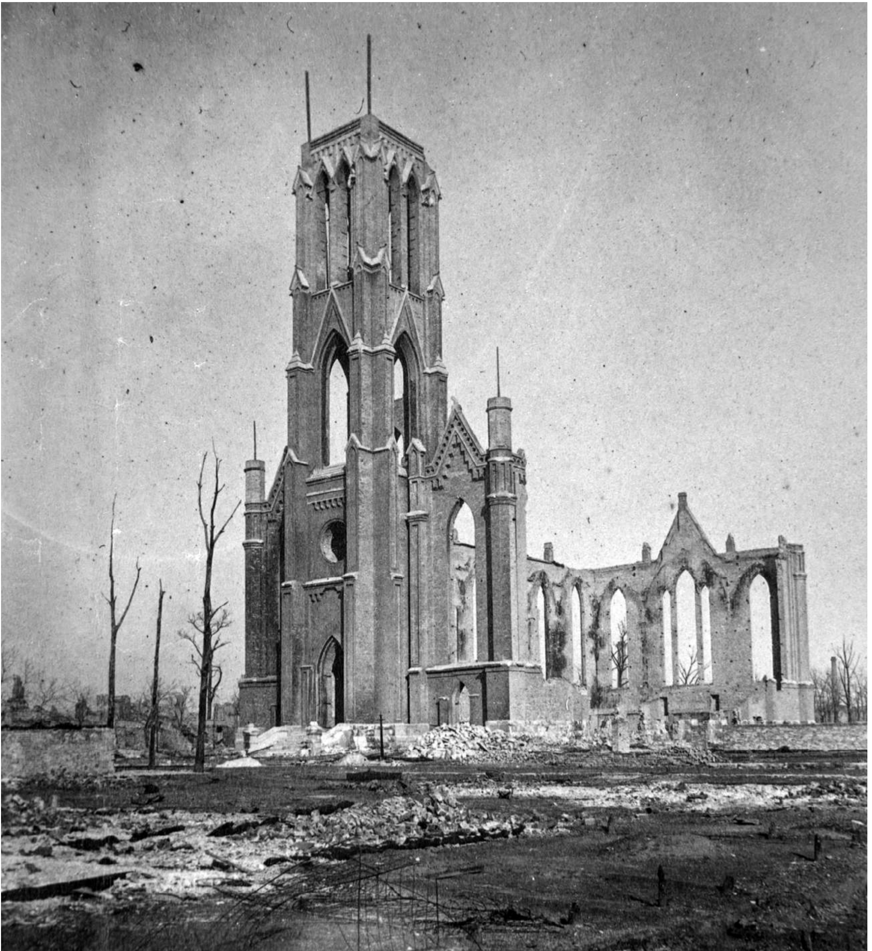
The remnants of Holy Name Cathedral after the fire.
