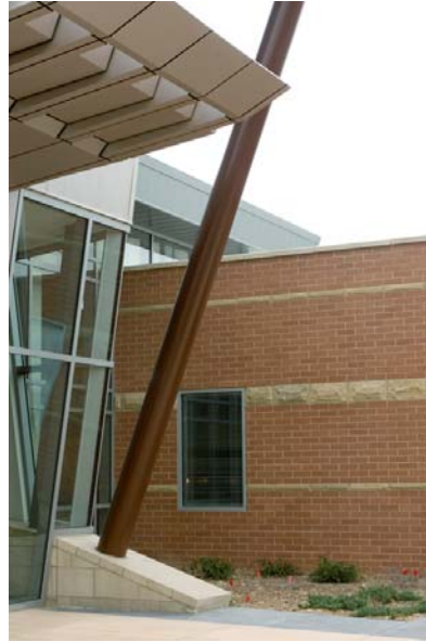
FIGURE 6 Local and regional materials—use of local masonry and other local materials.
