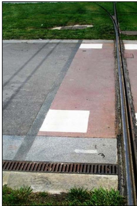
FIGURE 9 LRV dynamic envelope delineation, Barcelona, Spain (urban environment, median operation).
