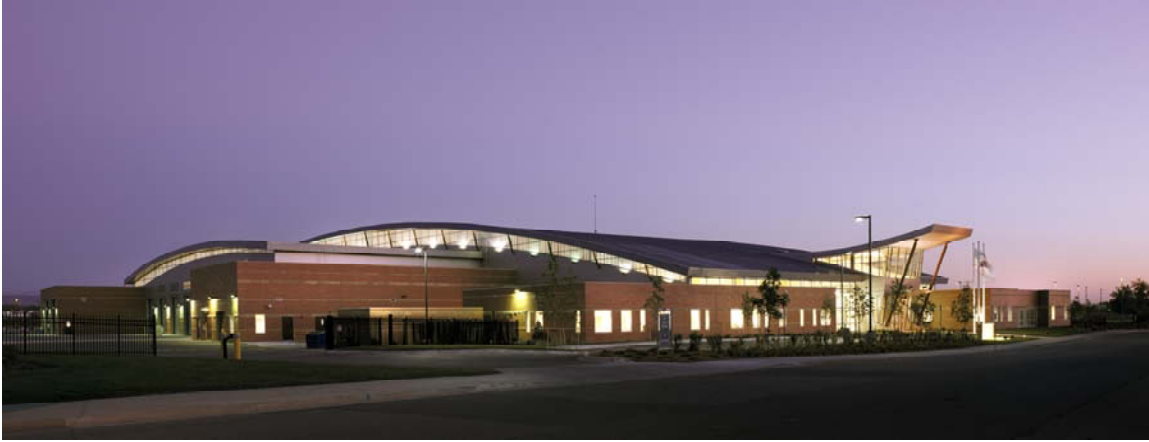
FIGURE 1 The curved roof form of the Elati Light Rail Facility is an example of form following function that complements its surroundings.
