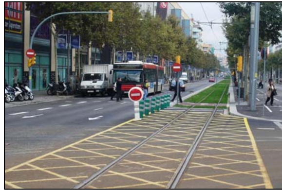
FIGURE 19 LRV envelope delineation (regulatory), Barcelona, Spain (urban environment, median operation).
