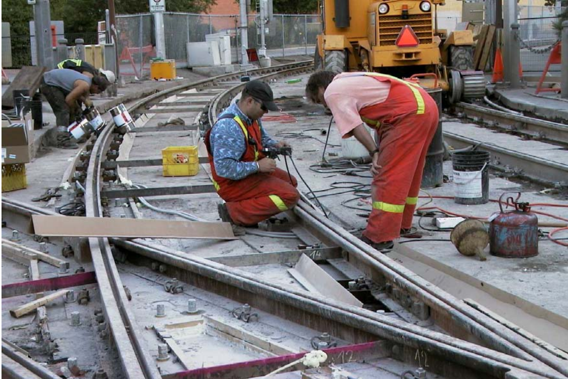
FIGURE 7 Calgary transit LRT staff replacing trackwork.
