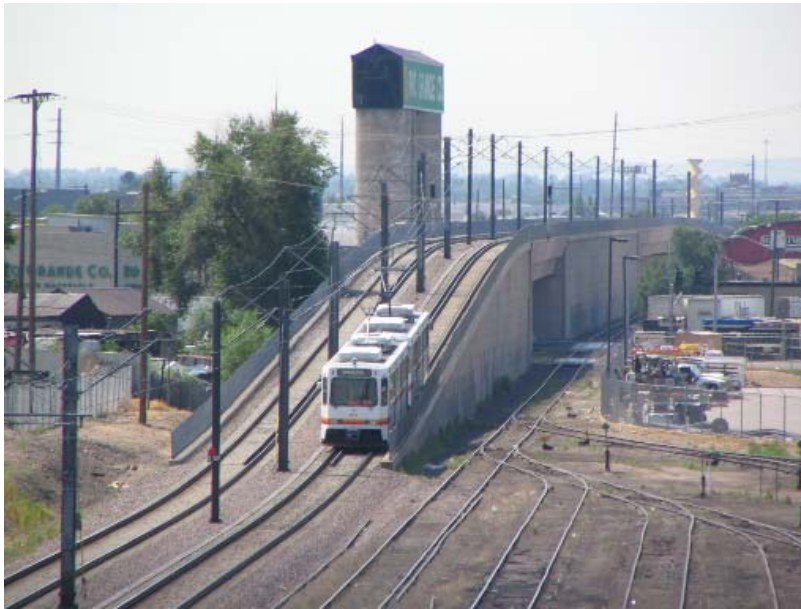
FIGURE 3 Light rail Santa Fe–Kalamath overpass.
