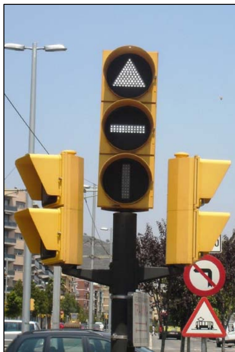
FIGURE 22 LRT signal indication (LRV Detected/Stop/Proceed), Barcelona, Spain.
