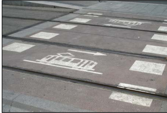
FIGURE 11 LRV directional striping (warning) on a one-way track, Barcelona, Spain (urban environment, median operation).
