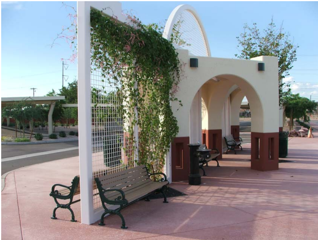
FIGURE 11 Passenger shelter at Gilbert park-and-ride facility. Source: TranSystems Corporation.
