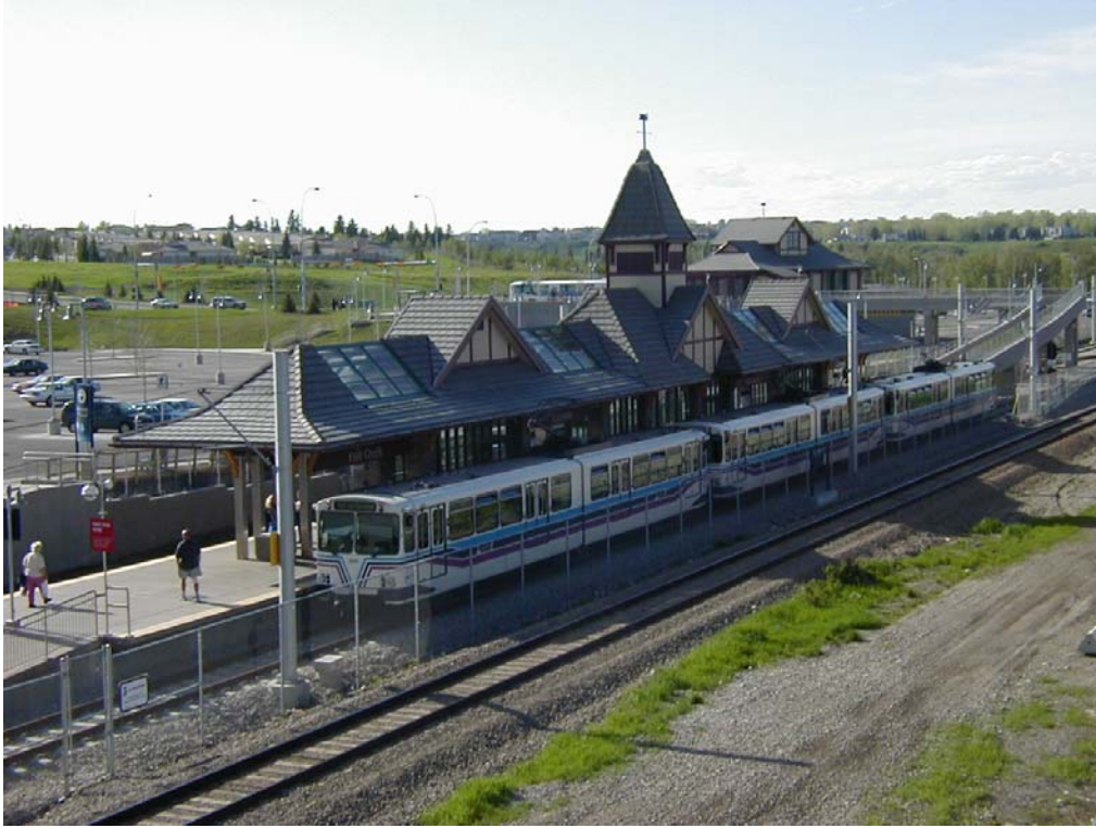
FIGURE 8 New Fish Creek Lacombe Station on south line in railway right-of-way.
