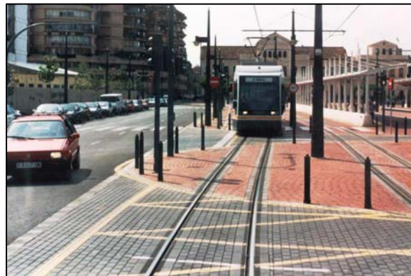
FIGURE 20 LRV envelope delineation (regulatory), Valencia, Spain (urban environment, median operation).
