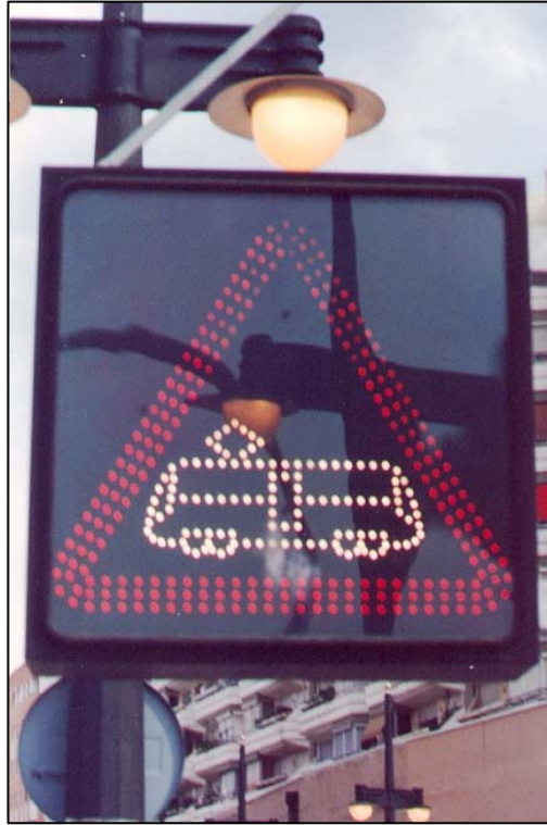
FIGURE 5 LRV-activated internally illuminated warning sign, Valencia, Spain (urban environment, median operation).
