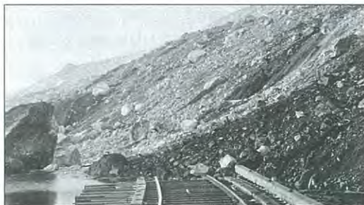
CPR main line buried by slide, 1903. (GAI)
