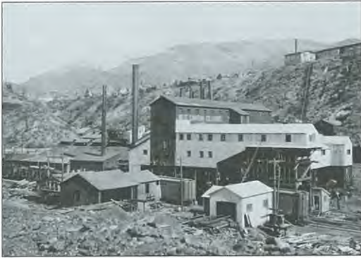
The Bellevue Mine. Note washhouse on the hill and the flight of steps leading down to the mine. (GAI)
