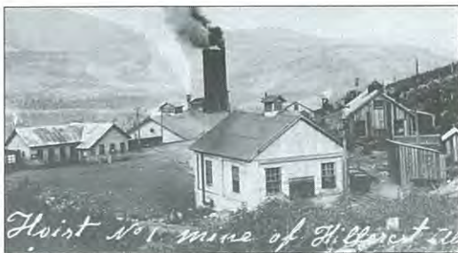
No. 1 Hoist House, Hillcrest Mine, before June 18, 1914. (PAA)
