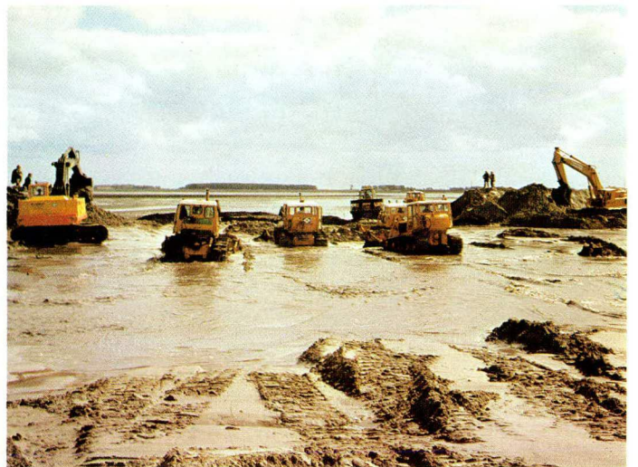
Closure of the ringdike at August 1977.
