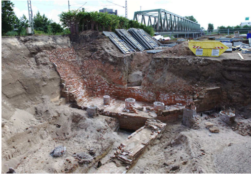
Fig. 3.7: Excavation of the rediscovered Stephanitorzwinger in Bremen, Germany.
