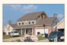
Foam sheathing and vinyl were lost on gable-end in Sunkist (Biloxi), Mississippi, just south of I-10. Massive water infiltration and damage to contents resulted.
