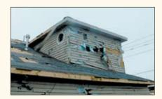
Plywood sheathing under badly battered vinyl siding remained intact on this wall.
