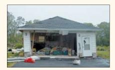
OSB wall sheathing fared well under lightweight vinyl siding compared to the non-structural wall sheathing materials shown here.
