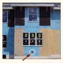
Some wall materials, such as the foam sheathing shown in the photo above, are susceptible to field damage. When holes are punched in the board during construction, any energy benefits from the foam sheathing are nullified by the resulting air infiltration.
