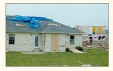
The nonstructural wall system of this two-story house offered little resistance to damage from flying debris and lateral forces.
