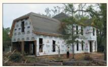
plete load path from foundation to roof, and the walls were fully sheathed with wood structural panels.
