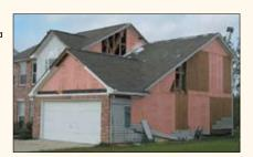
This home was in the same neighborhood as the above photo. Foam sheathing was inadequate to resist the wind pressures on the gable ends. Massive water infiltration and damage to home and contents resulted.
