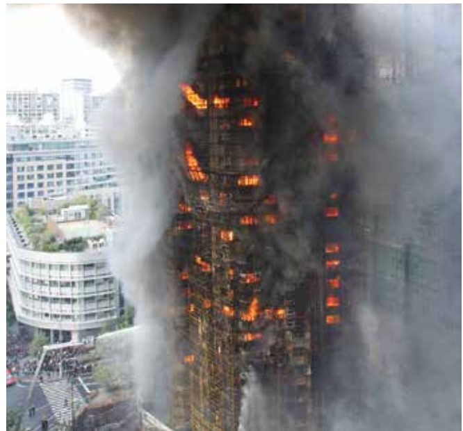
The severity of the Shanghai fire was partially a result of the use of urethane foam insulation, which aided in the spread of flame and smoke.
