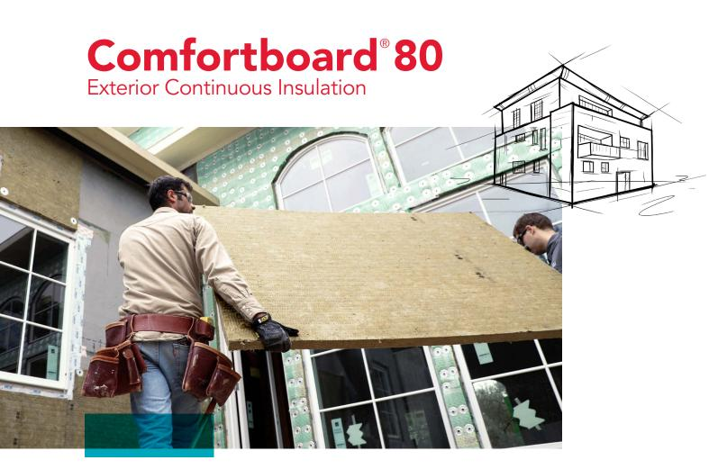
ROCKWOOL Comfortboard® 80 thermal insulated sheathing is a rigid stone wool insulation board designed for use as an exterior continuous insulation. Comfortboard® 80 does not produce smoke or propagate flames, keeping occupants safe and reducing property damage in the event of a fire. Vapor permeable, Comfortboard allows fast outward drying, keeping moisture out of your wall assembly.
