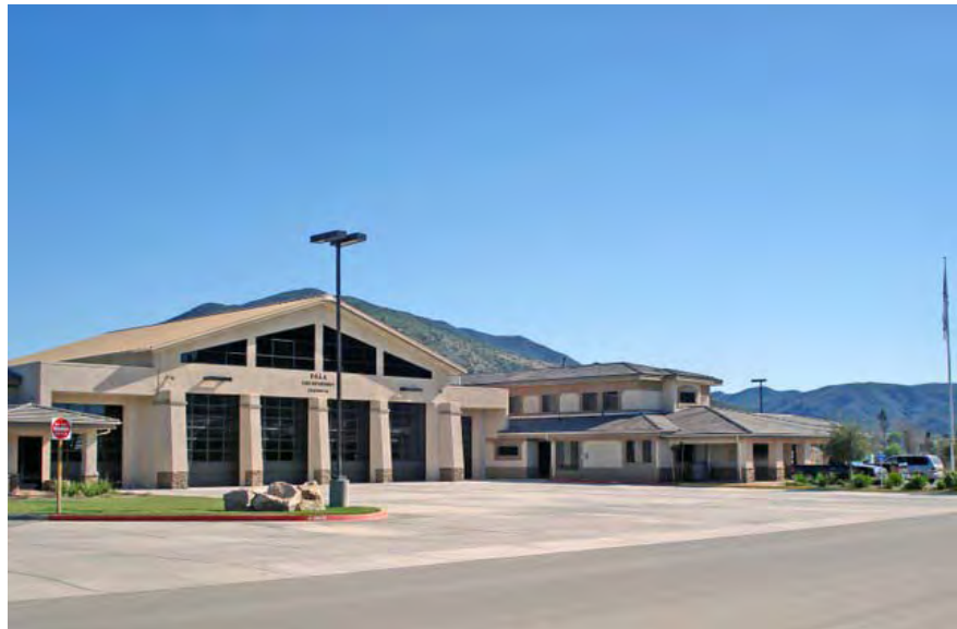
Figure 11. Pala Fire Station.
