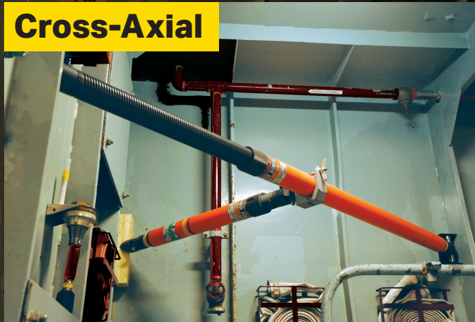
H-Type, can be used vertically or horizontally and takes moderate pressure (see table) as the pressure acts perpendicular to the load axis.
