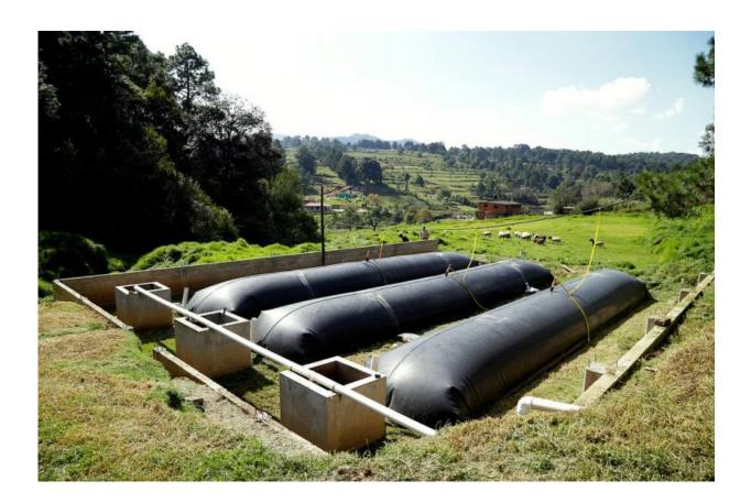
The principle of action of a cow's digestive system served as a model to create a container that receives organic waste, mostly livestock manure, where it is mixed with millions of bacteria to obtain natural gas consisting mostly of methane, called biogas, as well as a high-quality bio-fertilizer.
