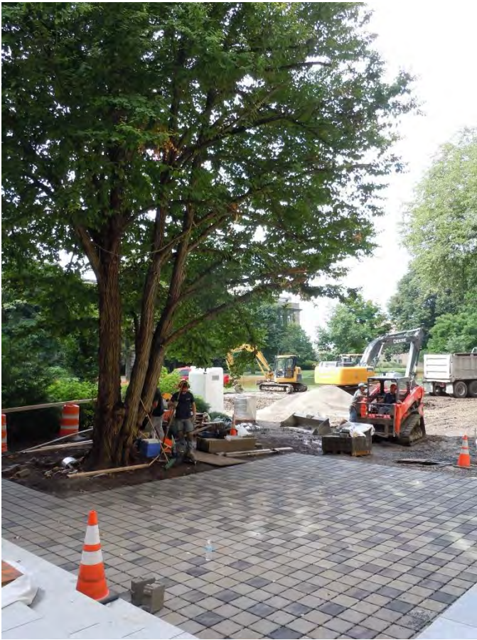
The nearly finished plaza space
