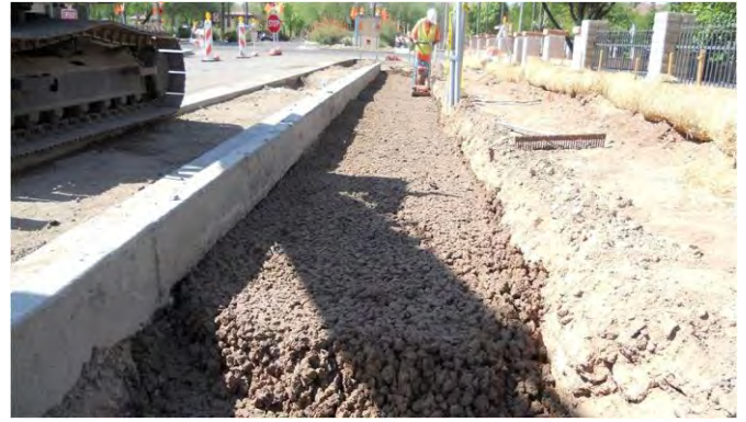
Compaction of CU-Structural Soil® during installation. For proper installation, CU-Structural Soil® must be compacted every 6 inches. Photo courtesy AZ Best, LLC
