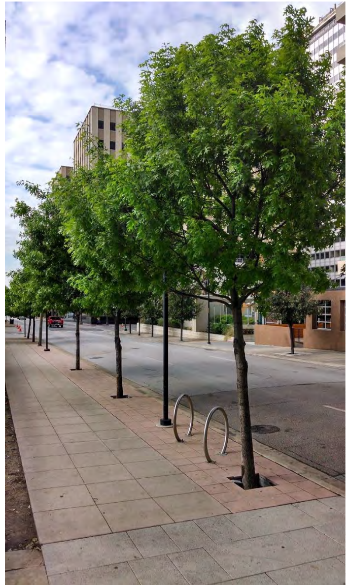
CU-Structural Soil® under this paved sidewalk provides these street trees with a continuous large volume of usable soil. Dallas, TX. Photo courtesy Minick Materials Company
