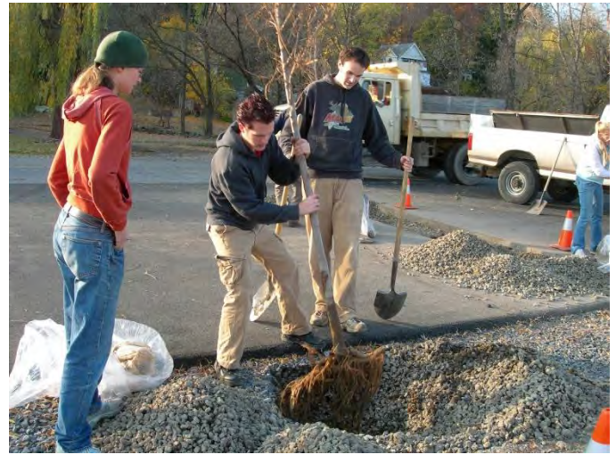
Planting the bare root elms directly into CU-Soil® in 2005
