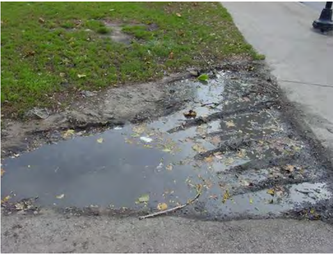
On this traditional lawn corner the turf has been worn away by automotive traffic. This traffic compacts the soil and limits drainage, essentially drowning out the grass
