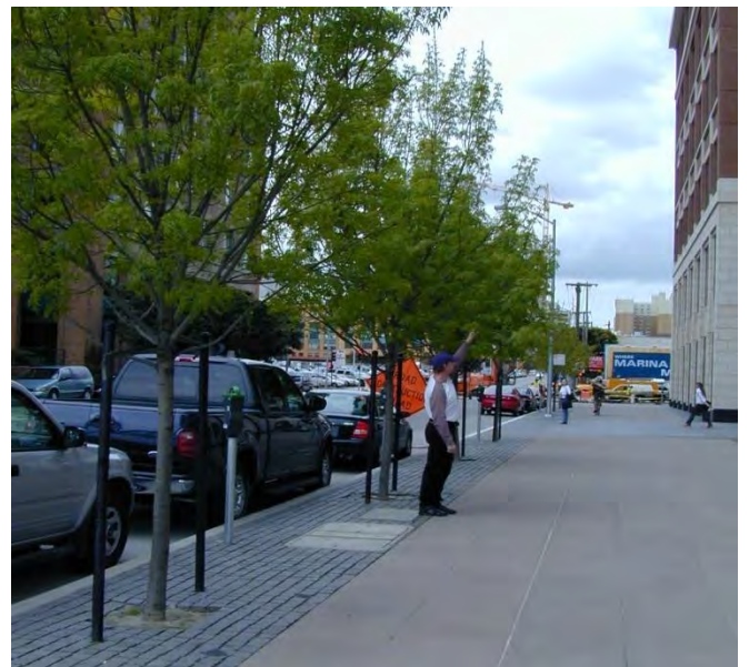
This installation uses cobble pavers with porous joints as the covering of a continuous trench of CU-Soil®.
