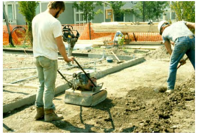
Compaction of soil in preparation for pavement
