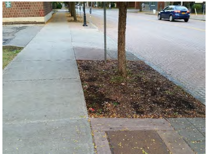
A typical tree pit on W. State Street. The colored concrete sections correspond with the extents of the CU-Soil® volume.
