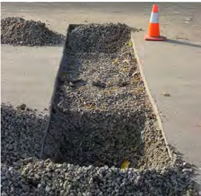
The saw-cut planting bed with holes dug in the CU-Soil® for tree planting.
