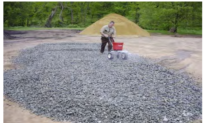
Gelscape® Tackifier being applied to uniformly sized crushed stone. Photo courtesy Amereq, Inc.
