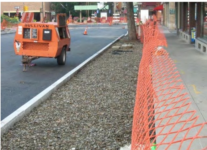
Installation of the new sidewalk on a base of CU-Soil®. This picture also shows an existing mature tree
