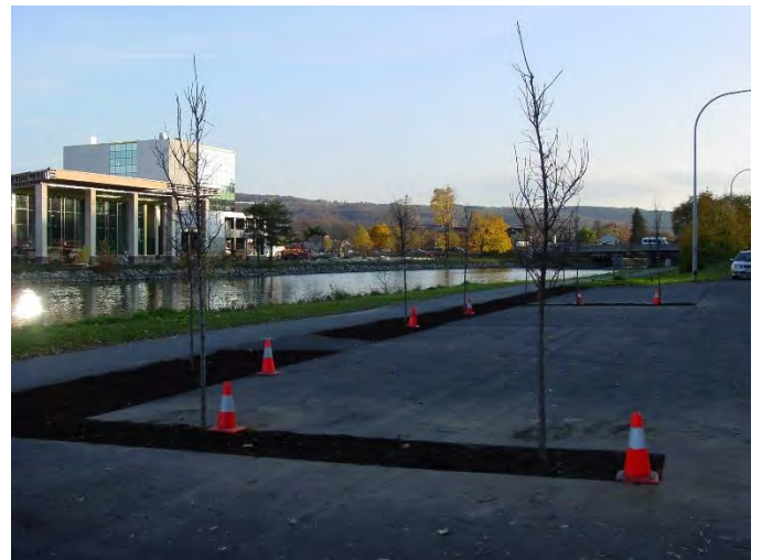
The finished parking lot
