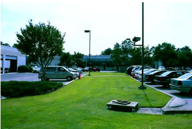
The finished installation. Photo courtesy Southpine, Inc.
