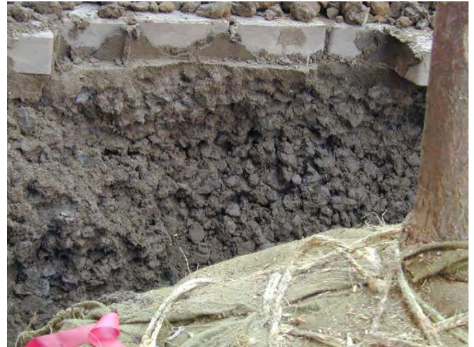
Closeup of CU-Structural Soil® after installation
