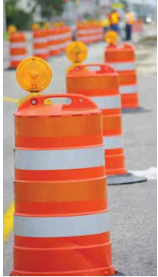
Barricade lights at construction site.
