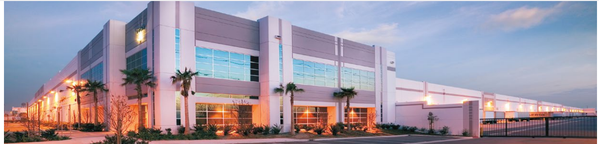
Prologis Kaiser Distribution Center, Inland Empire, California.
