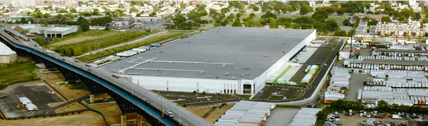
Prologis Pulaski Distribution Center, Jersey City, New Jersey.
