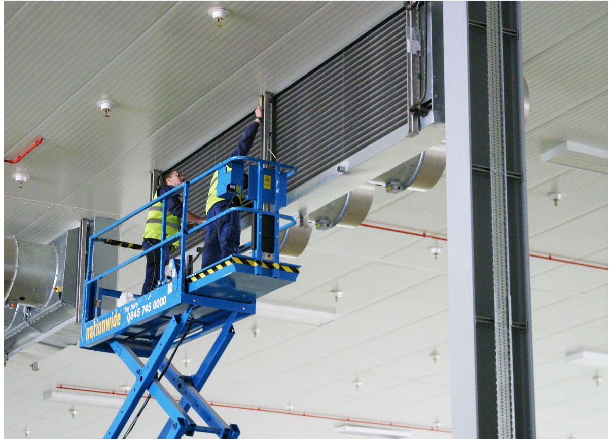
Prologis Park Pineham, Northampton, UK.
