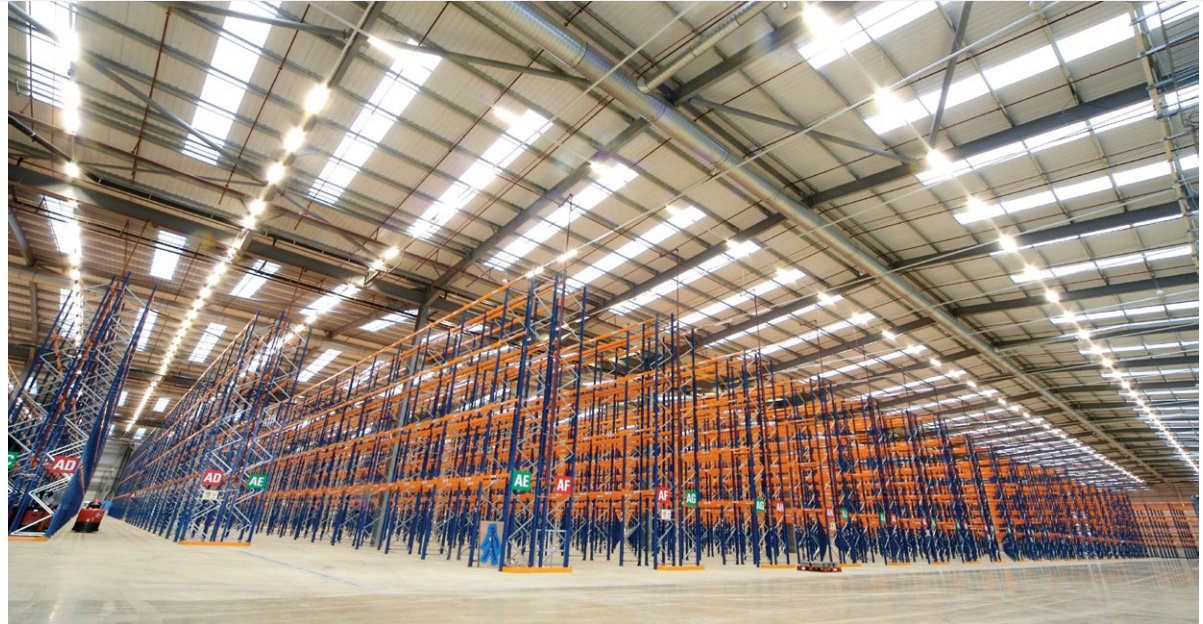
Prologis Park Pineham, Northampton, UK.
