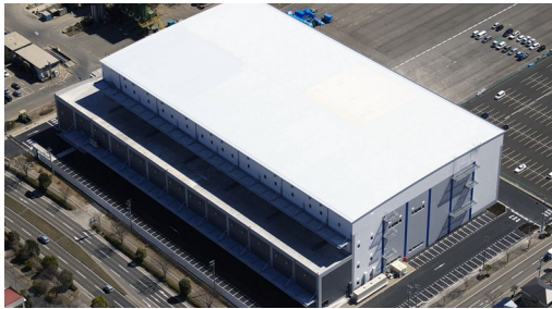
Prologis Park Tagajo Distribution Center
