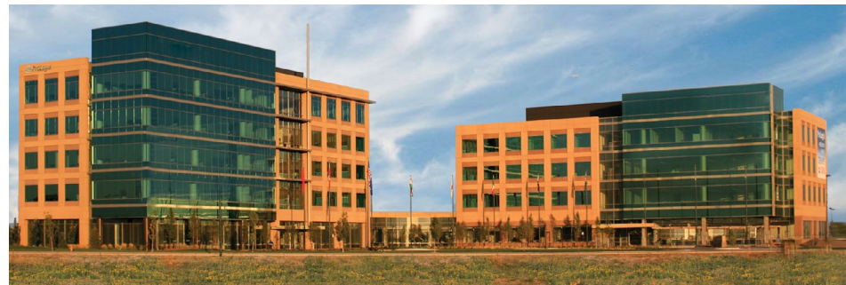
Prologis Denver Operational Headquarters
