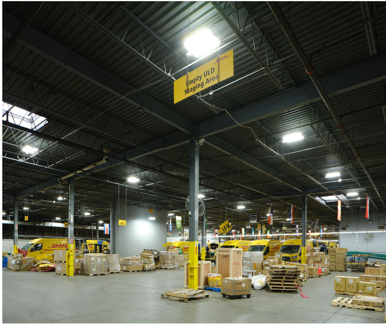
LED lighting installation, Prologis Ports Newark, New Jersey.
