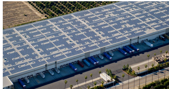
Solar installation at LEED Silver-certified Prologis Park Redlands, California.
