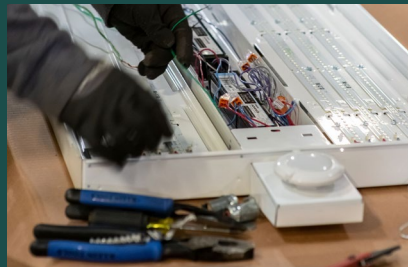
Installation of energy-efficient fixtures from our Prologis Essentials LED lighting program
