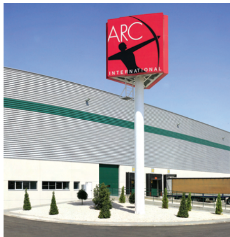
PROLOGIS ZARAGOZA SPAIN
