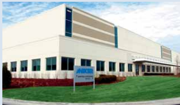
Anixter International Facility at ProLogis Park 294 (Chicago, IL – US)
