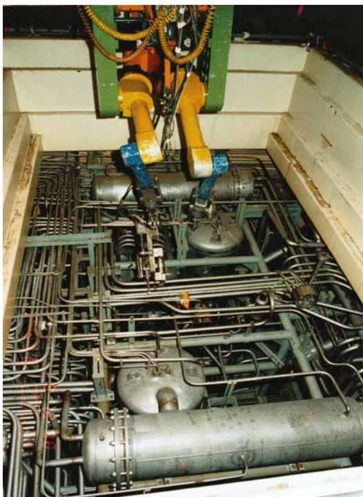
Figure 2: Remote dismantling of the HLLW evaporator cell
