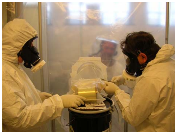
Fig. 2: Bag-out of material contaminated in the incident from within the protective enclosure As it was decided to retain safe 3 for future use, this phase of the clean-up also involved the decontamination of safe 3 itself and the disposal to active waste of the contaminated removable parts (trays and sliding mechanism). Permanent markings have been applied to safe 3 to indicate that the
