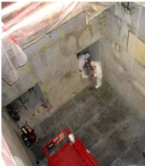
Figure 3: HLLW evaporator cell after removal of the pipe penetration blocks
