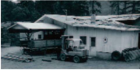
First facility near Grants Pass, Oregon c.1970
