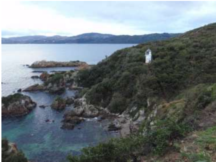
Figure 83: Matiu/Somes lighthouse and landing bay
