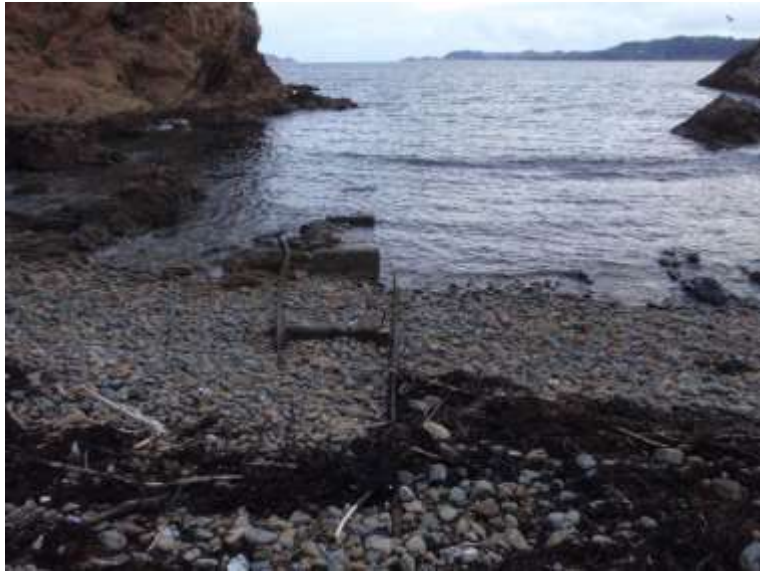
Figure 84: Visible extent of rails and concrete supports in landing bay
