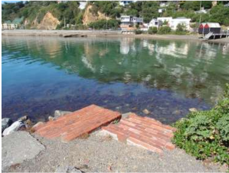
Figure 99: Brick rubble used in reclamation at northern end of Balaena Bay. Looking south across bay.
