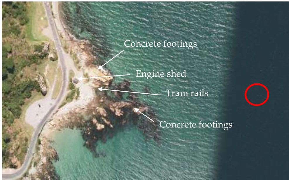
Location of submarine cable remains indicated in red, Point Gordon, image from Google Maps, 2012
