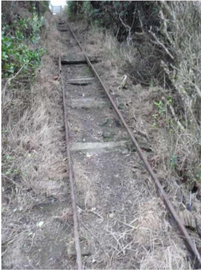
Figure 86: Tramway rails leading to lighthouse
