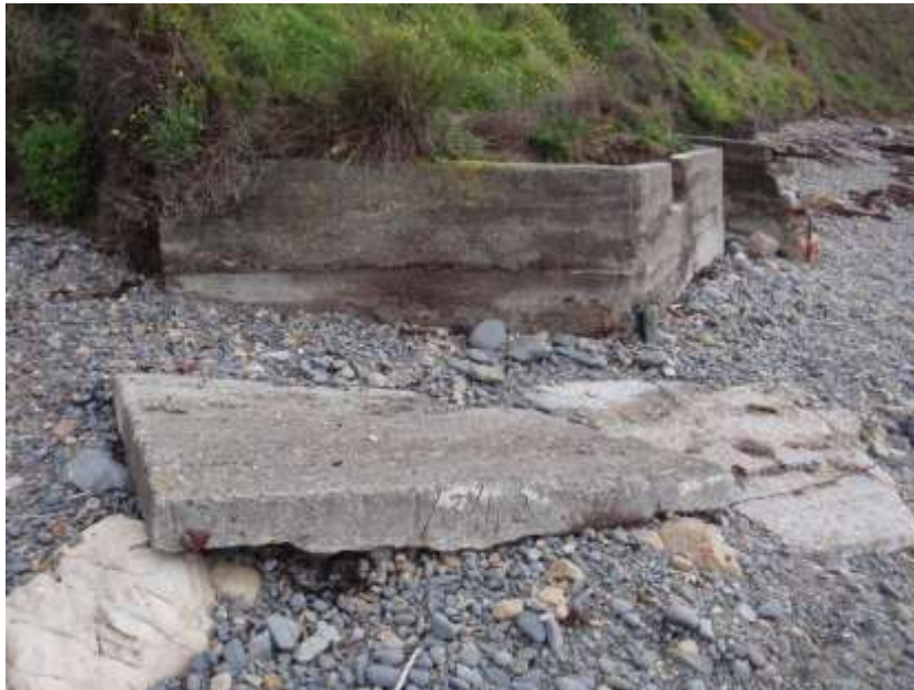
Home guard position viewed from northeast. Note date incised into concrete 1/3/42
