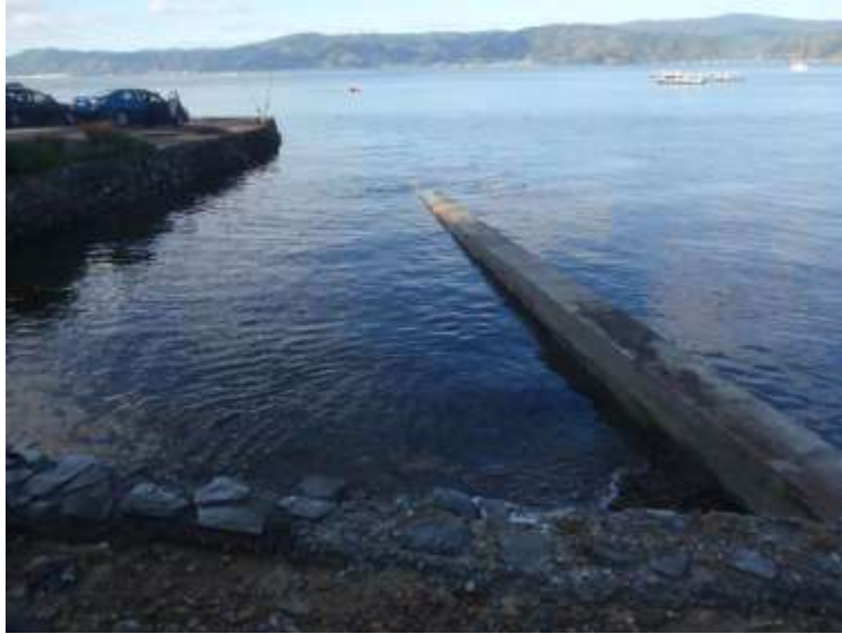
Figure 82: Location of Mahanga Bay wharf as viewed from the shore
