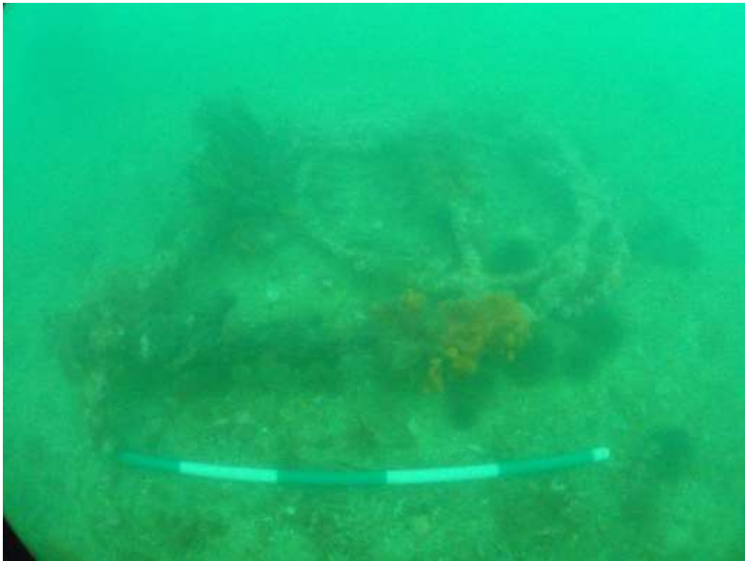
Tangle of cable on the seabed off Point Gordon likely to be from either the 1890 minefield linked to Point Gordon or the WWII minefield controlled from Worsler Bay
