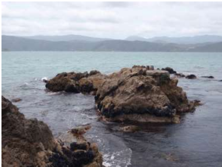
Figure 77: Concrete and timber remains on rocky outcrop at Point Gordon
