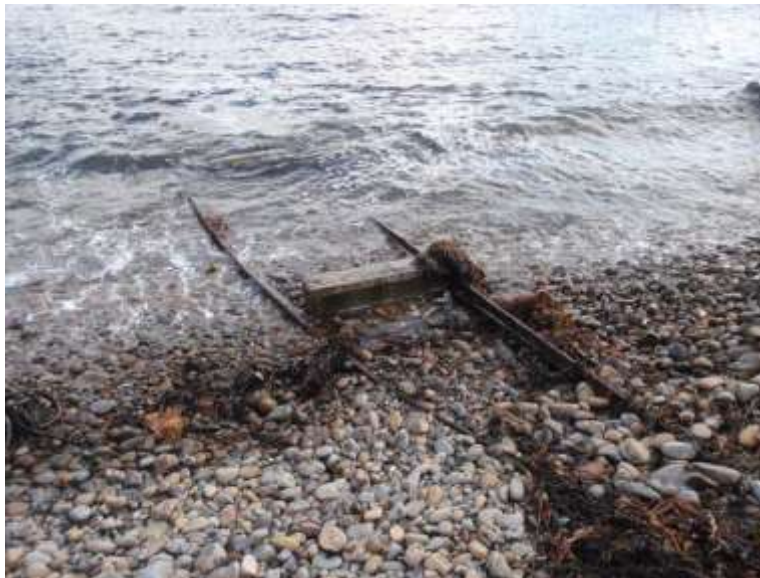
Figure 85: Close up of remains of landing
