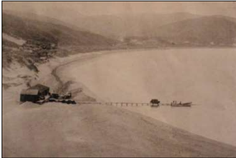
Figure 88: Transferring goods between jetty and long boat (reproduced from Castlepoint historical committee publication, 1948)
