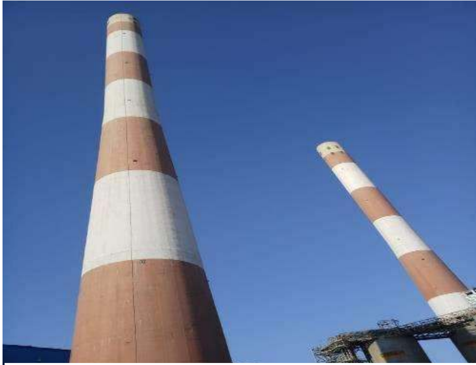
Tall Stack (Ht 220m) attached with Boilers
