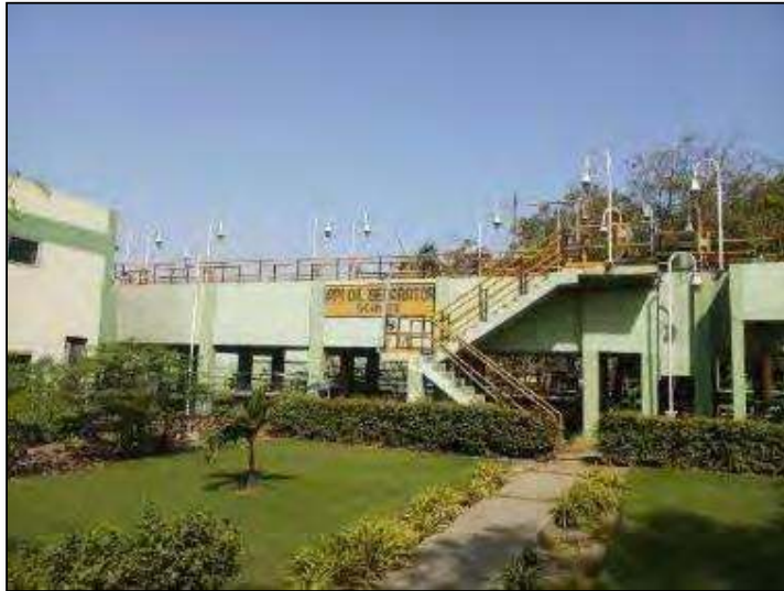
Oil Separator Unit
