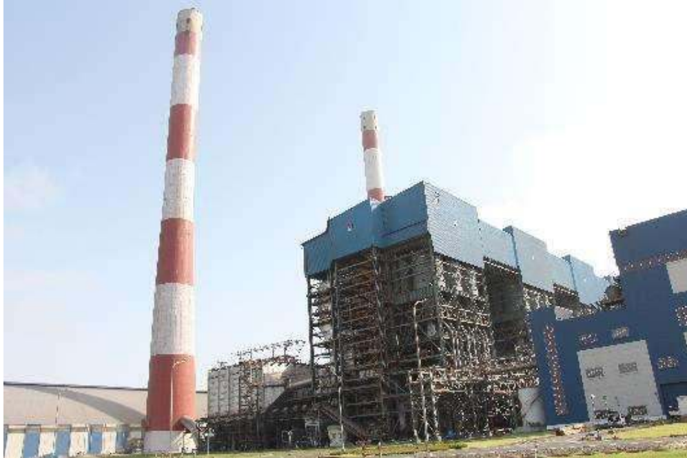
Stacks (Ht 220m) attached with Boilers
