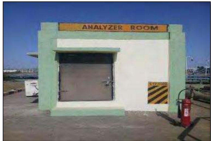
Analyzer room for Continuous Effluent Monitoring System
