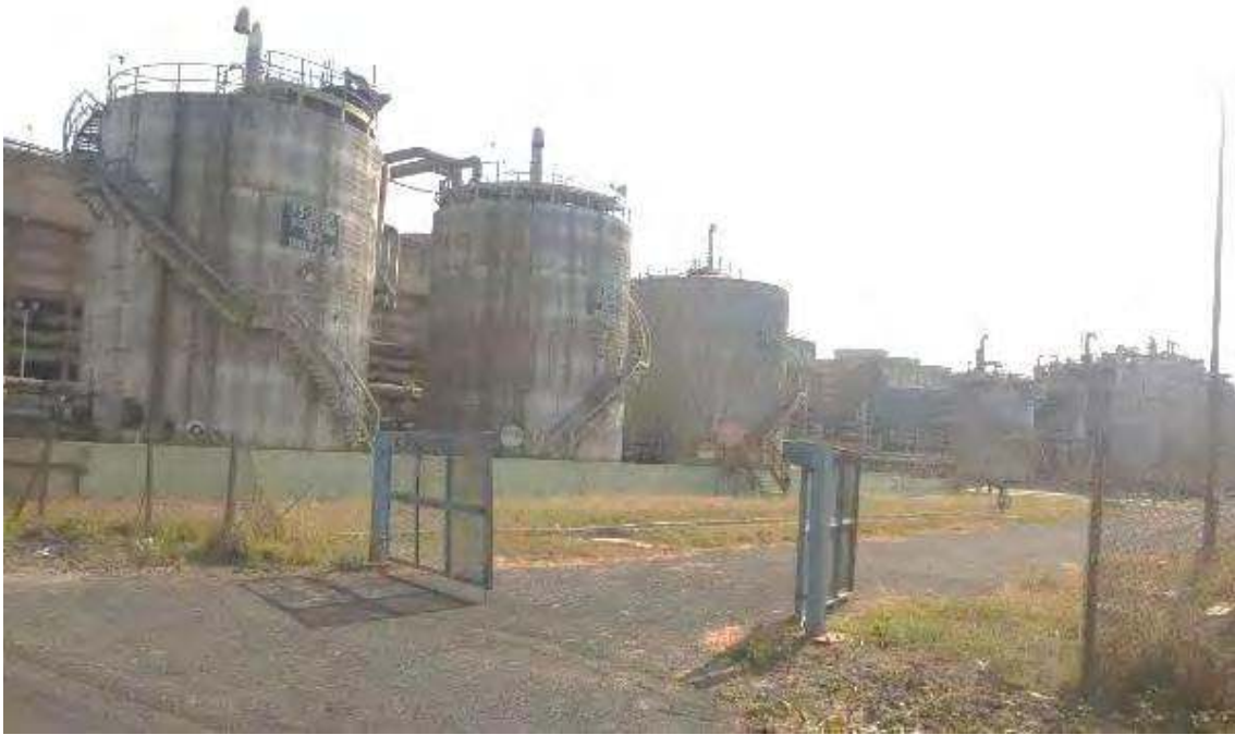
Photograph of PTA Storage Tanks
