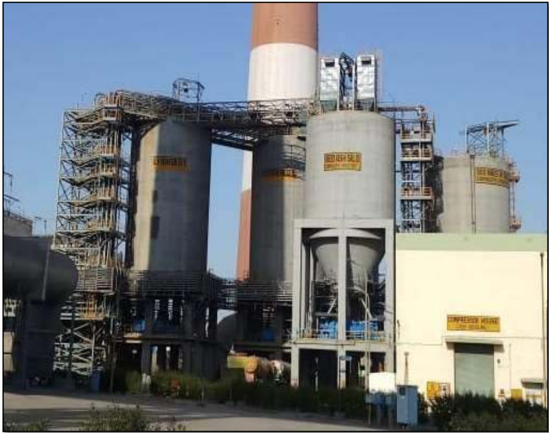
Photograph of Fly Ash Silo
