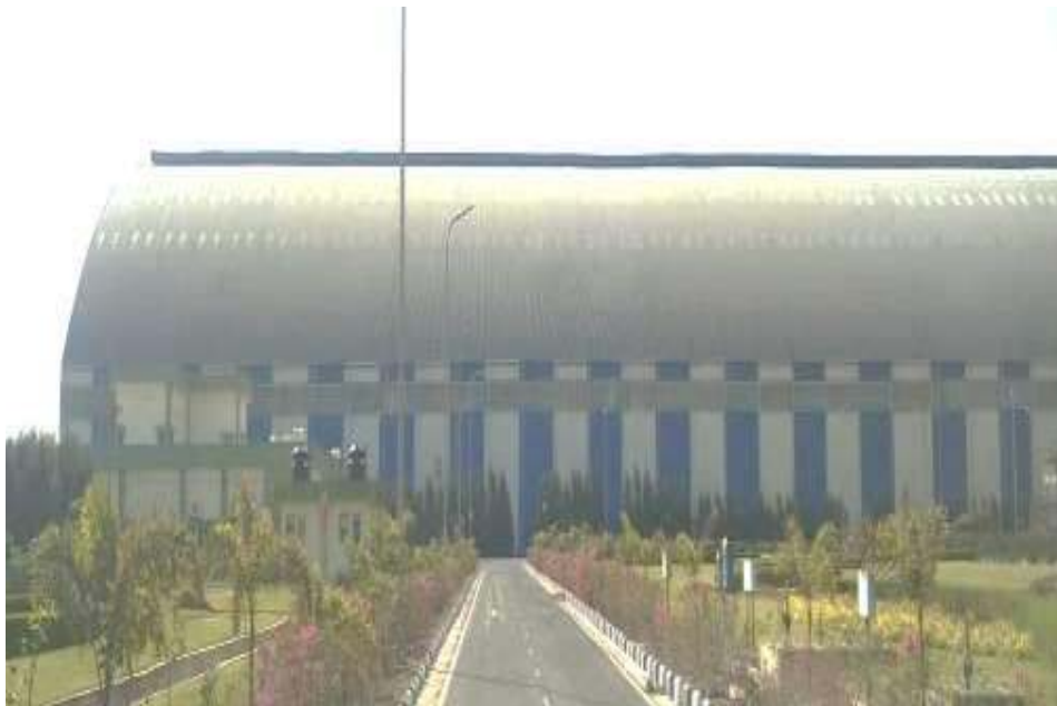
Fully Covered Coal Storage Area
