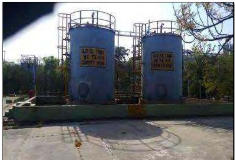
Slop Oil Storage Tanks
