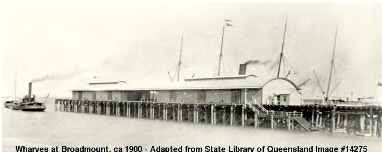
Figure F: Broadmount Wharf
