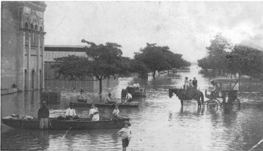
Flooding, East Street, Rockhampton, 1918.
