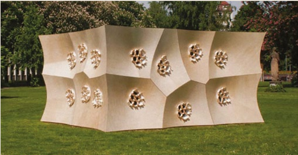
Image: The project HygroSkin – Meteorosensitive Pavilion explores a novel form of climate responsive architecture, its intricate wooden designs autonomously opening and closing in response to changes in the weather. © ICD University of Stuttgart.
