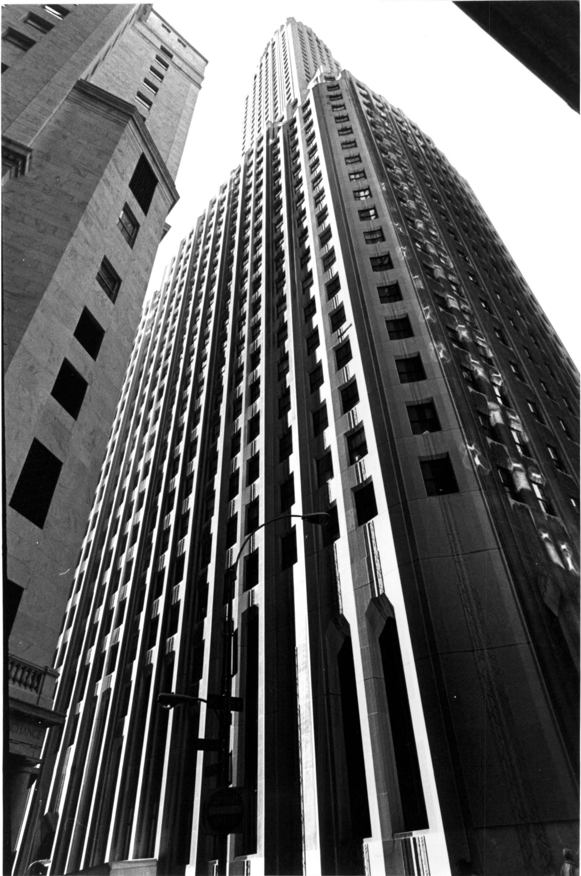
1 Wall Street Building , 1 Wall Street, Manhattan Wall Street facade Photo: Carl Forster
