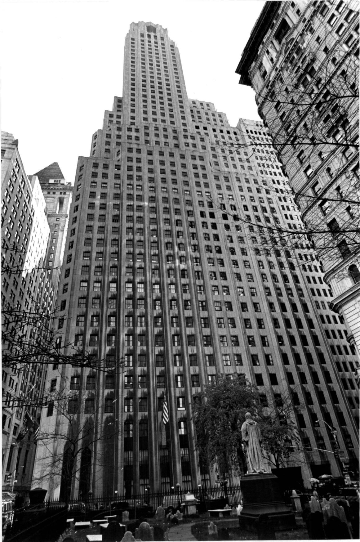
1 Wall Street Building , 1 Wall Street, Manhattan Broadway facade Photo: Carl Forster
