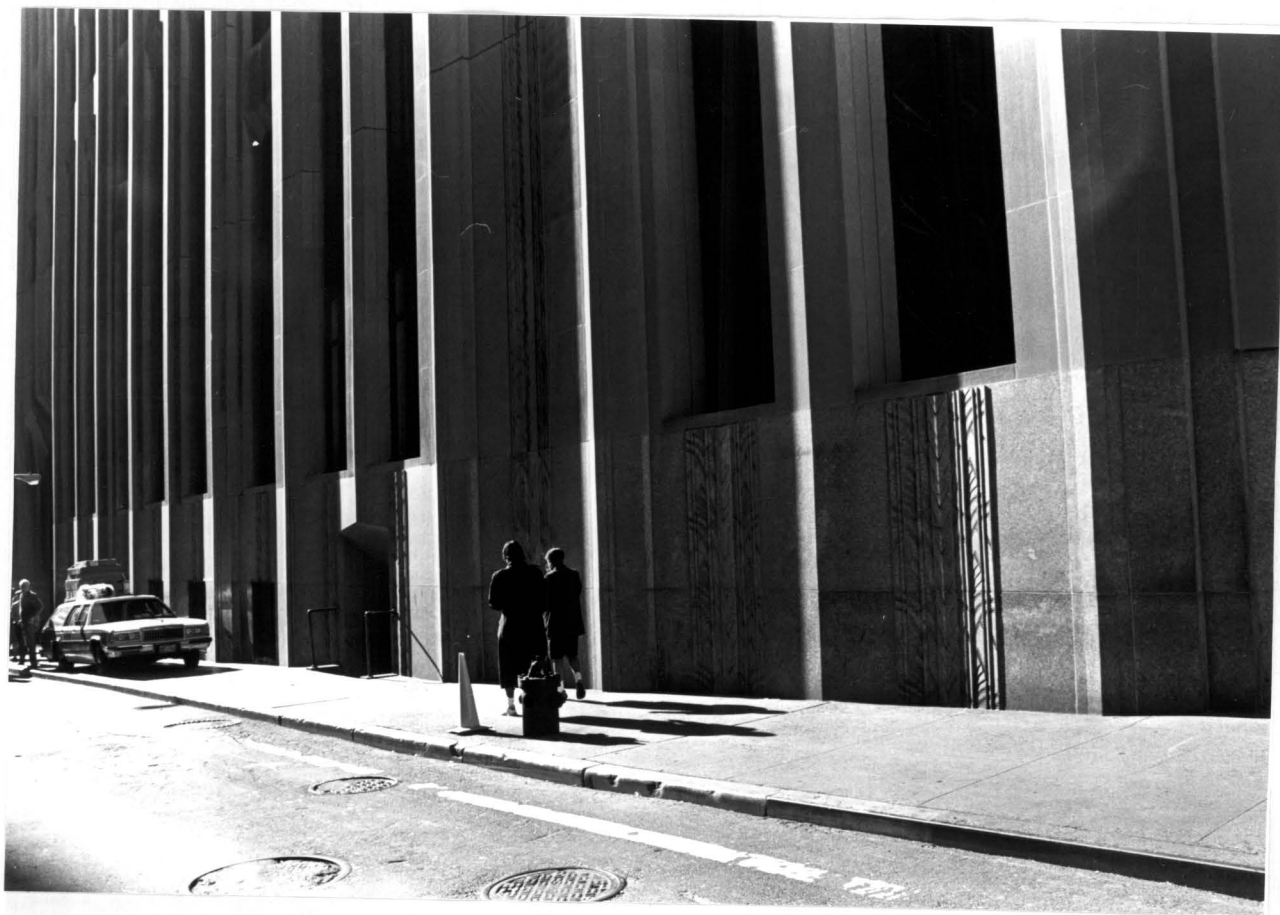
1 Wall Street Building Base, New Street facade Photo: Carl Forster
