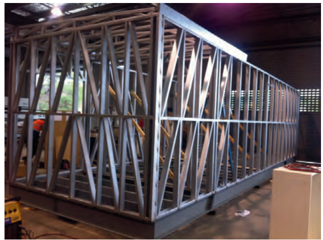
Images courtesy of Emerson Network Power
