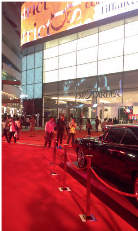
The EmQuartier now boasts a smart low-voltage network.
