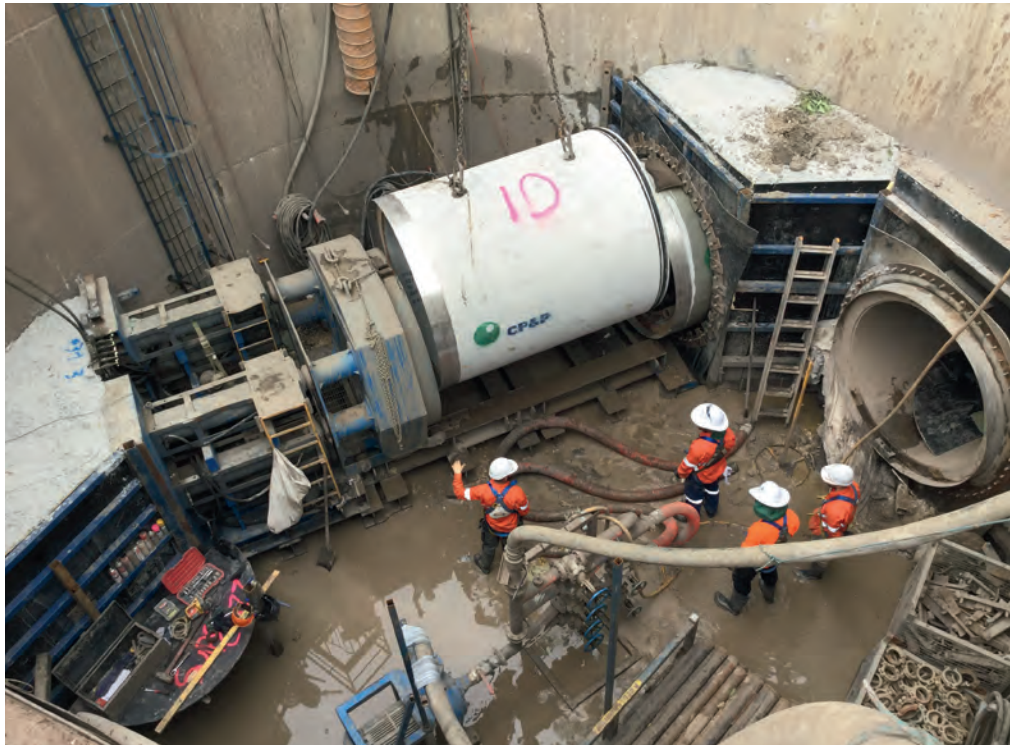
Microtunnel pipe installation inside caisson.
