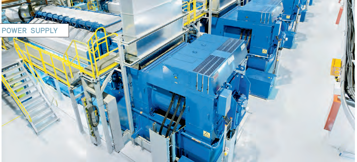
Figure 1: The alternators in grid-support plants must be designed to accommodate the thermal and mechanical stresses caused by the need to ramp up and down in response to variable renewable generation on the grid. Shown is power generation equipment with separate generating units at the Kiisa power plant in Estonia.
