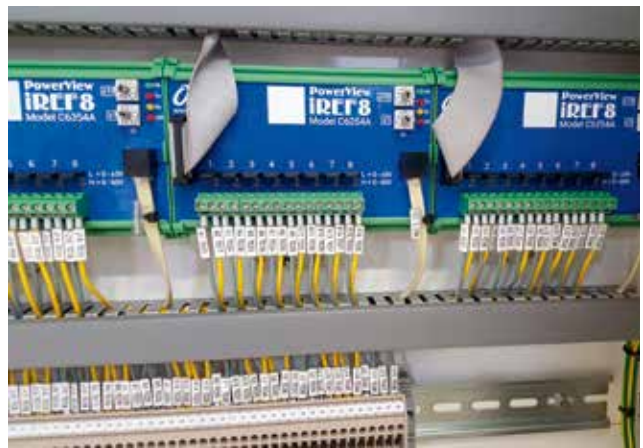
Omniflex's PowerView iRef8 monitoring unit.
