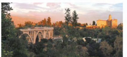
Pasadena's iconic Colorado Street Bridge is illuminated by the city's famous sunset glow. visit PASADENA
