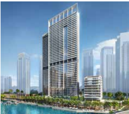
Dubai Creek Harbour Palace Hotel & Residences, UAE
