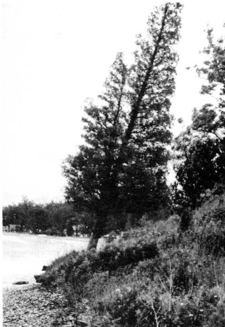
Figure 10. This tree used to be at the top of the bluff before the land beneath it slumped.
