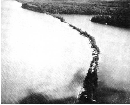
Figure 15. Bay barriers are important natural erosion protection features.
