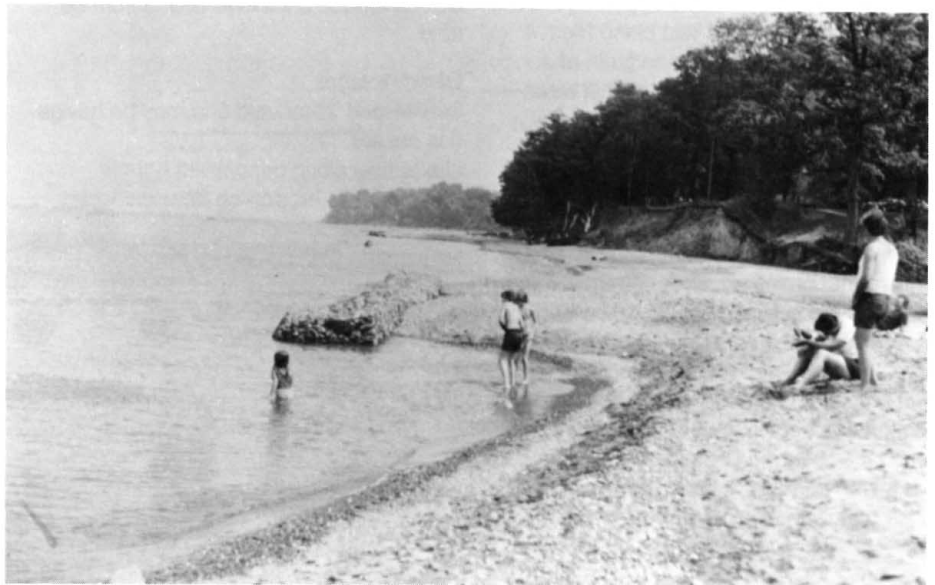
Figure 28. Gabion breakwaters can be used in protected or sheltered locations where winter ice is not a factor and where wave energies are fairly low.
