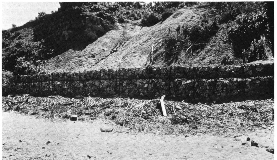
Figure 21. Gabion bulkheads are suitable in areas with no ice or when used above the ice line.
