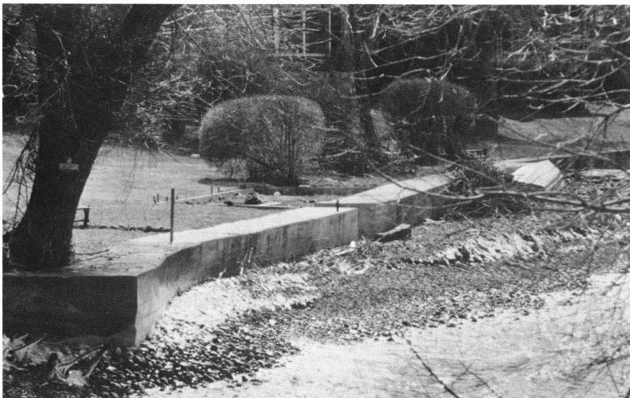
Figure 16. Cast-in-place concrete bulkheads resemble seawalls.
