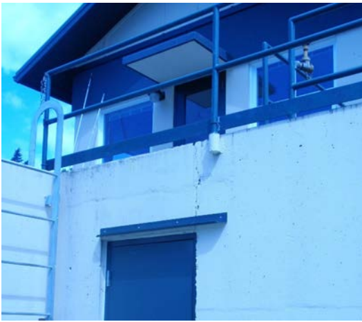
Figure 4-1. Filters Exterior South Wall
