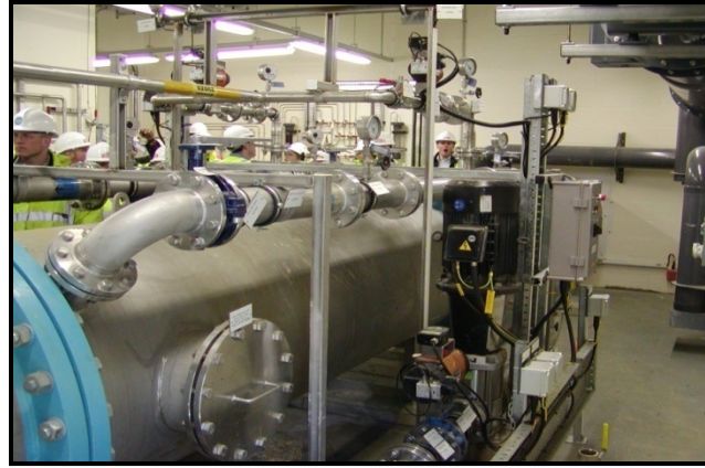
Sidestream Ozone Injector
