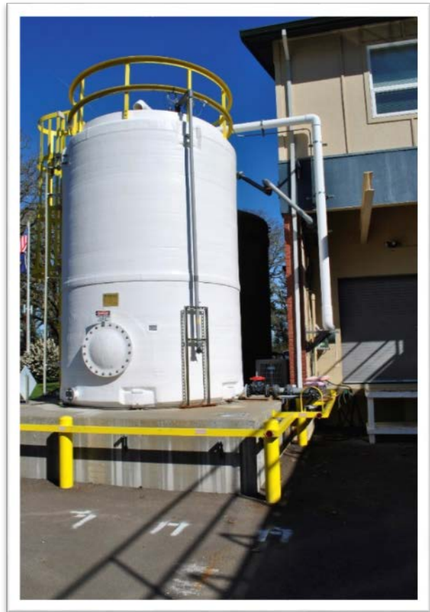
Figure 6-16. Hypochlorite Tanks
