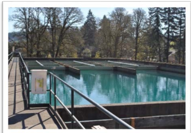
Figure 6-8. Sedimentation Basin
