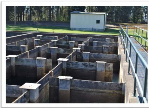
Figure 6-7. Hydraulic Flocculators
