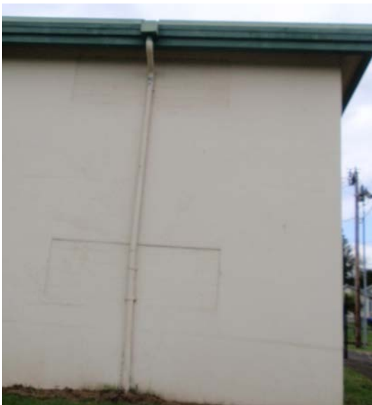
Figure 4-7. DSPS Exterior Wall Corner
