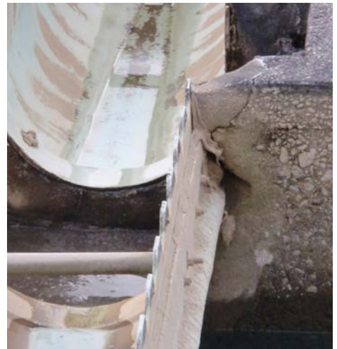
Figure 4-6. Launder Trough Anchorage
