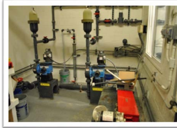
Figure 6-14. Hypochlorite Feed System
