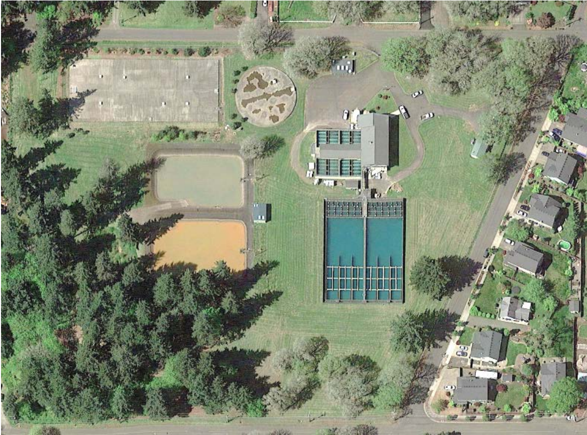
Figure 2-1. SFWB WTP Aerial Photograph
