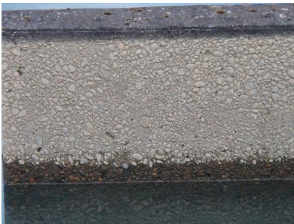
Figure 4-5. Flocculation/Sedimentation Basin Interior Wall
