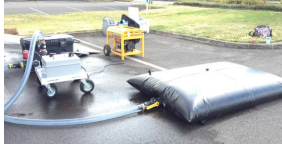
Figure 6-20. Photos of Distribution System Manifolds
