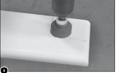
Using the proper size hole saw bit, drill holes in the sill at the center points you marked.
