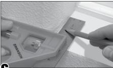
Hold a combination square to the bull nose corner as shown. Locate the tangent point of the corner radius. Measure the distance.
