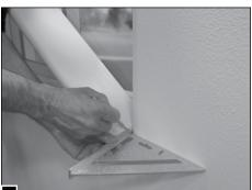
Insert sill into the window opening at an angle with the back of the sill butt up against the window frame. With a square against the face of the wall, mark the depth of the window opening on the sill.
