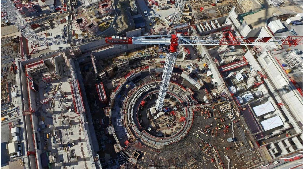
ITER under construction (Photo: ITER organization)
