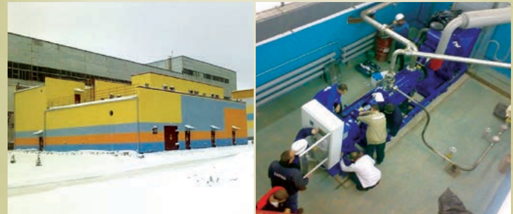
Figure 3.2. Additional independent system of emergency feeding to the steam generators at power units №1, 2 of RNPP
