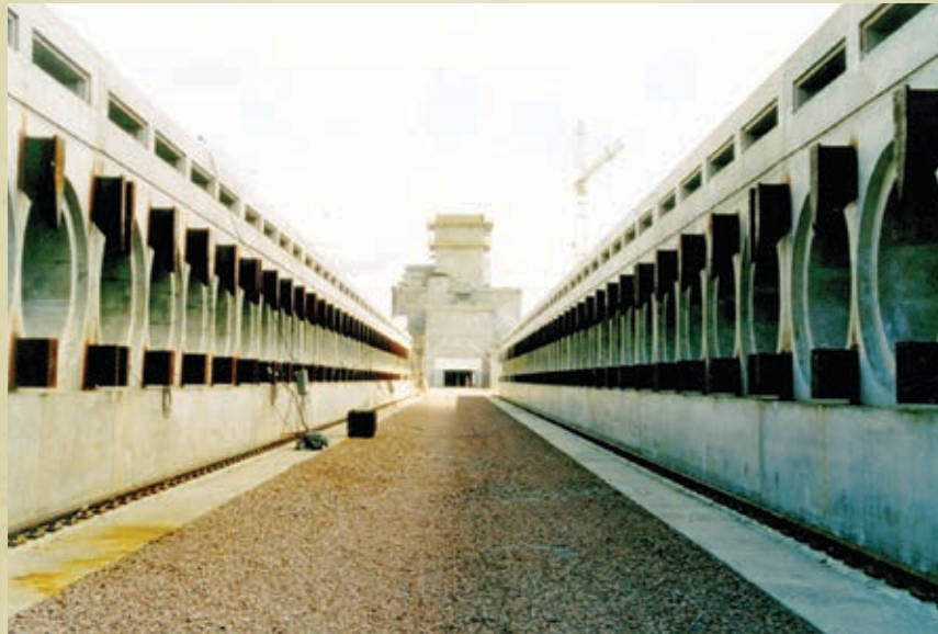
Figure 4.9. Concrete storage module in the fuel storage area of ISF-2
