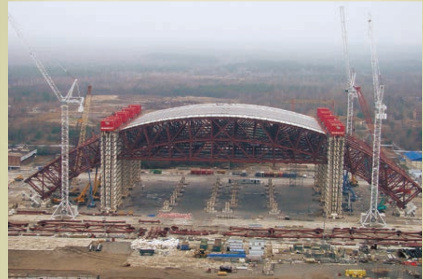
Figure 4.1. First lift-up of NSC metallic constructions
